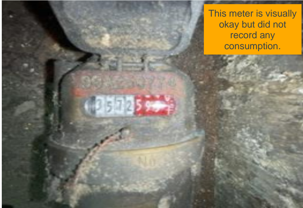
This meter is an older meter, estimated to be installed in 1987. It's visibly okay and is confirmed to not be recording consumption.
